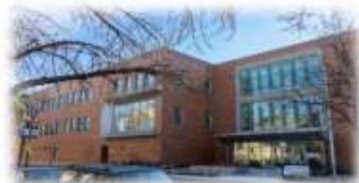
Thomas Waters Elementary School Brick in Architectural Awards 2021
